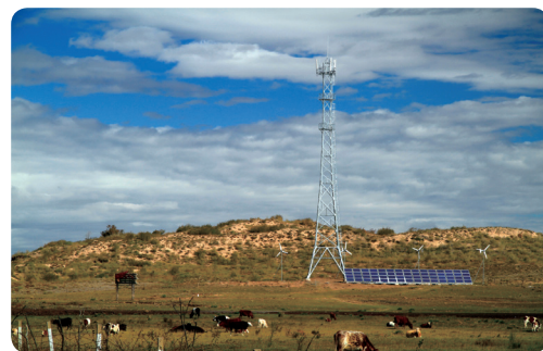
Solar-powered base stations in Inner Mongolia, China
